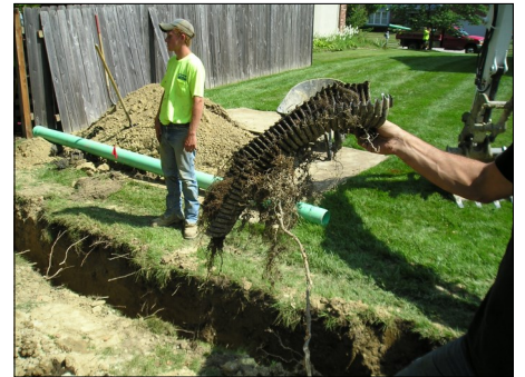
Tree roots can plug up drainage pipes— large and small. Willow and birch tree roots can be particularly aggressive. Photos: Hamilton County Surveyor's Office
