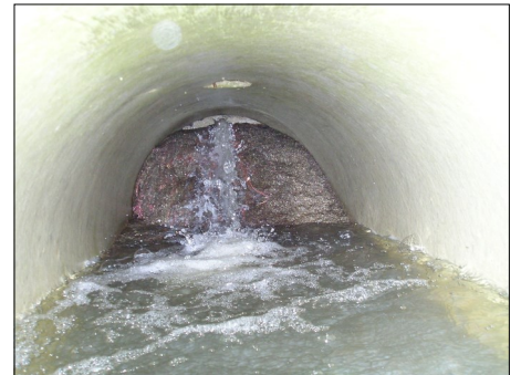
Tree roots can plug up drainage pipes— large and small. Willow and birch tree roots can be particularly aggressive. Photos: Hamilton County Surveyor's Office
