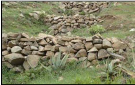
Rock Grade Stabilization Structures
