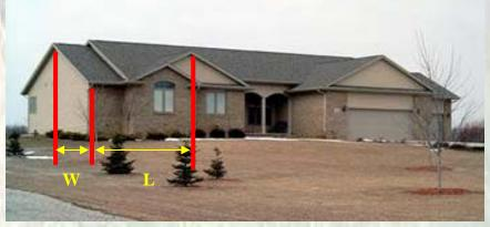
Example: This house has a simple roof. There is a gutter that collects the roof water from the peak and ridge on the front of the house. You would need to measure from gutter to peak which is "W" and from the end of the house to the ridge line which is "L". The drainage area is W x L. Take your measurements in feet to get an answer in square feet.
