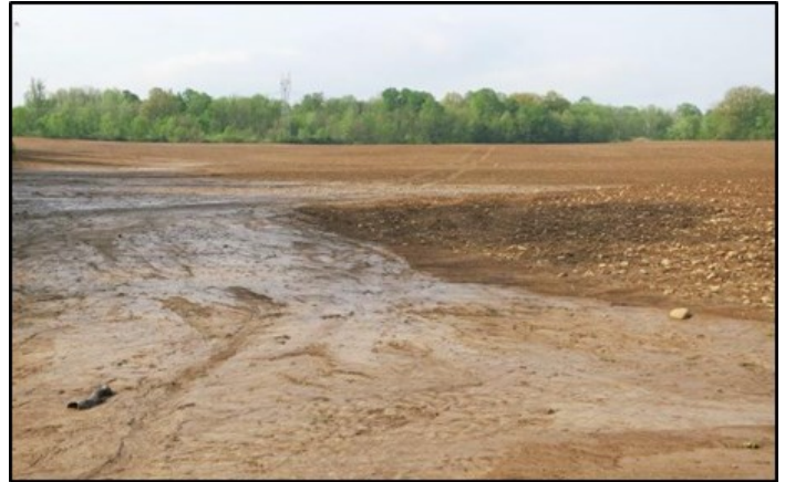
Sediment bars will need to be shaped with a dozer.
